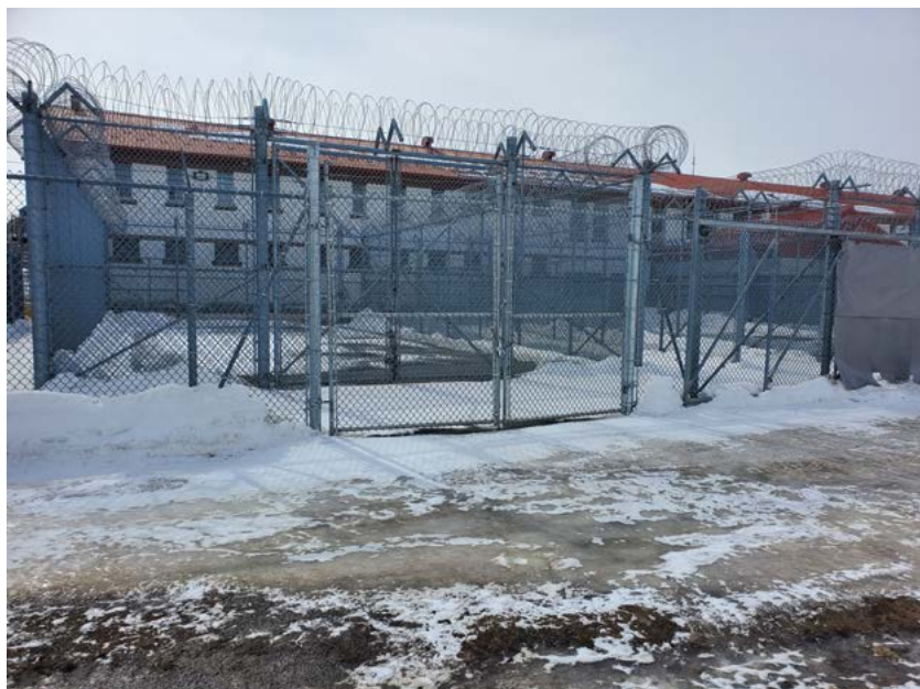
The medical isolation unit yard at the Federal Training Centre
